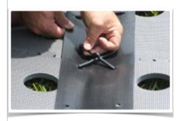
The floating plant mats consist of puzzle cut mats held together by nylon connectors. These mats may be assembled in any size or shape
