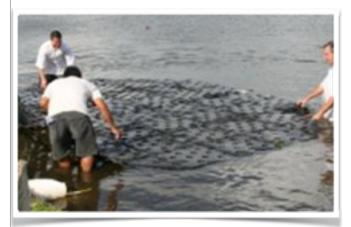
After the mats are connected, plants are inserted into pre-cut holes. The plants may be any species of emergent aquatics. The mats can be attached to anchors or shoreline stakes.
